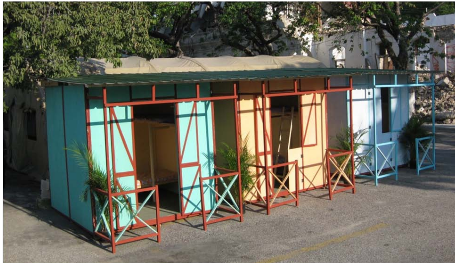
The living quarters constructed for the girls living at Camp Oasis.
